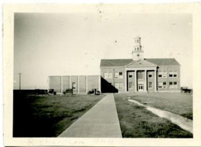
Construction of South Wing, c. 1929
