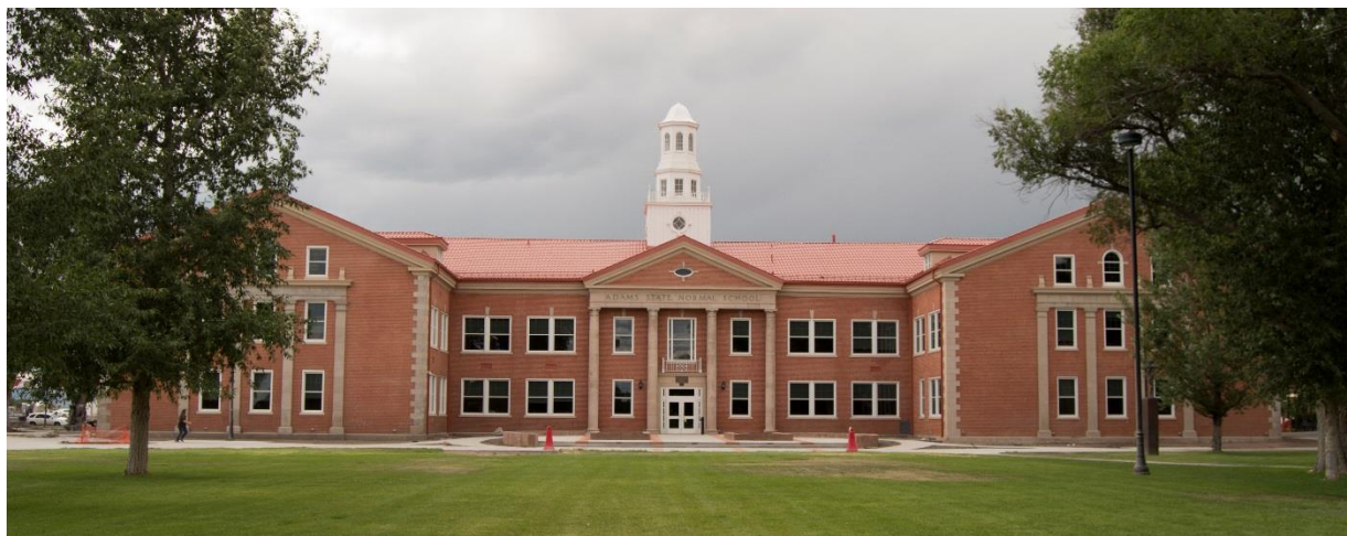
East Elevation, July 2015
