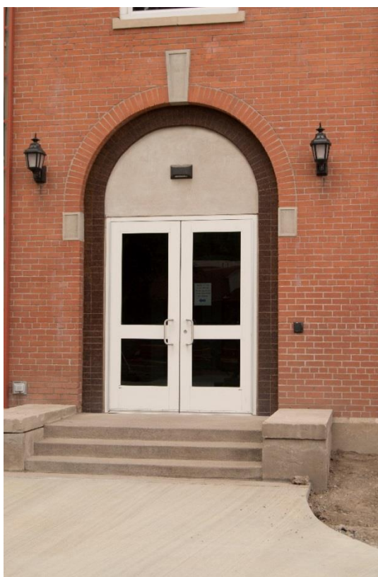
Side entrance, July 2015
