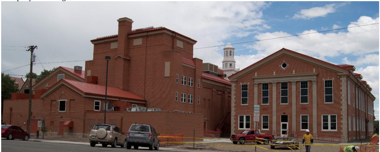
Southwest Elevation, July 2015
