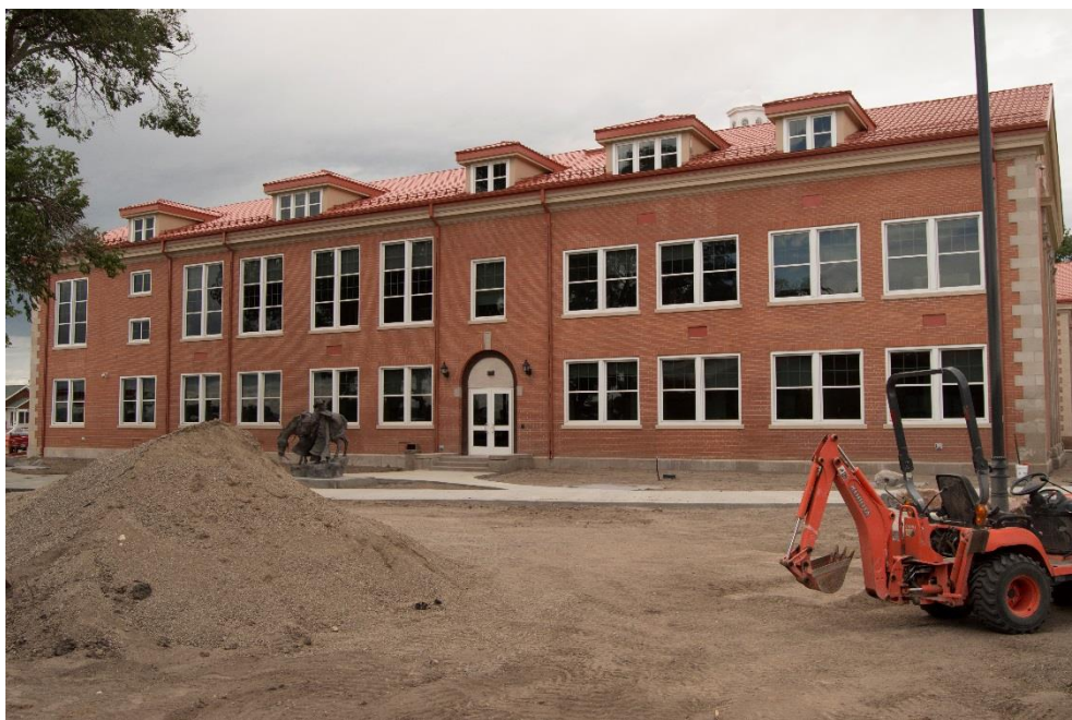
South Wing, July 2015
