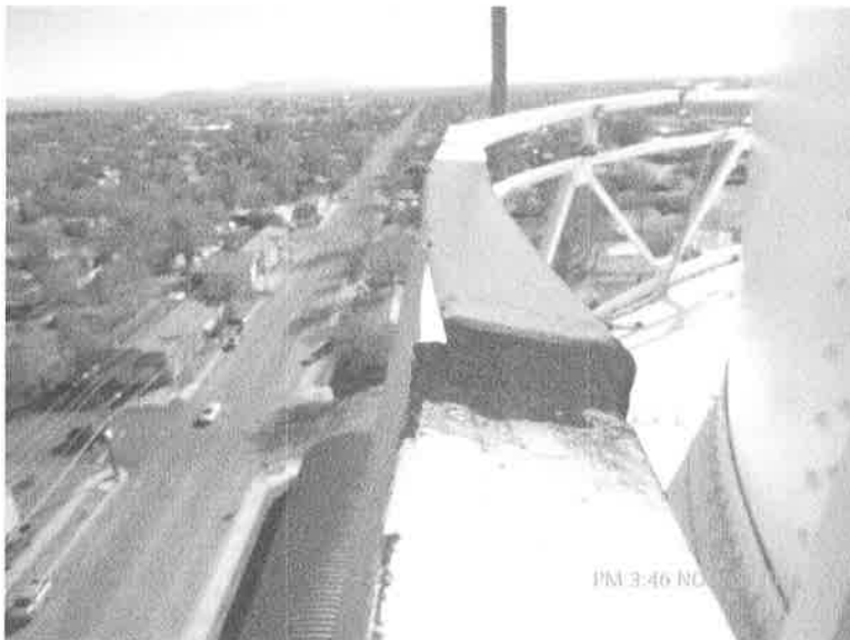
Existing Upper Handrail-Rusting Poor Layup
