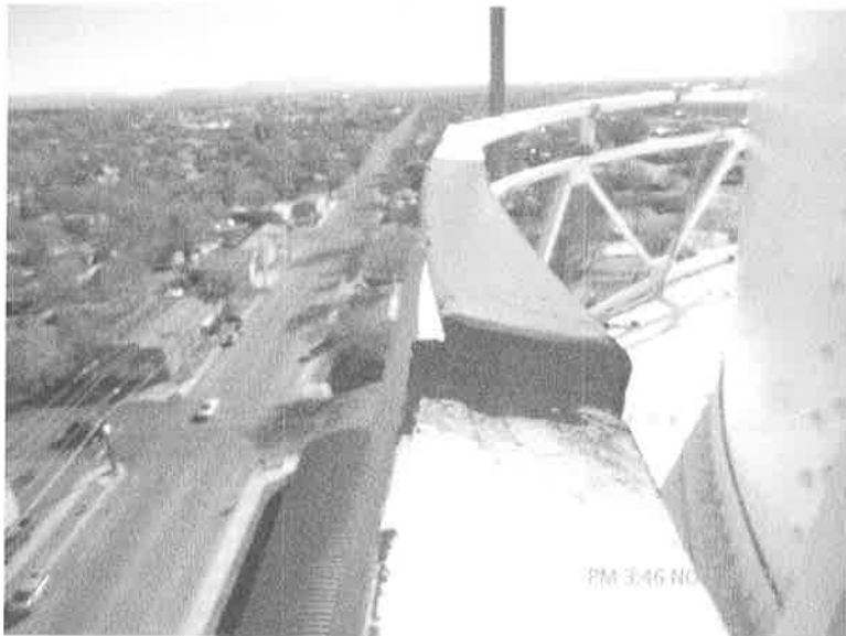
Existing Upper Handrail-Rusting Poor Layup
