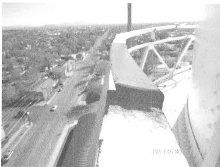
Existing Upper Handrail-Rusting Poor Layup
