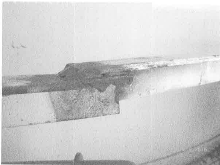
Existing Upper Handrail-Rusting Poor Layup
